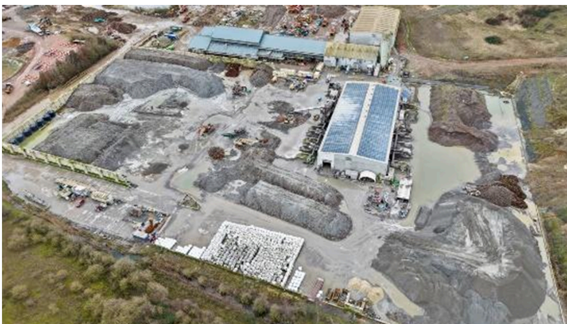
Figure 3. Incinerator bottom ash processing site, Cambridgeshire, UK. 7
