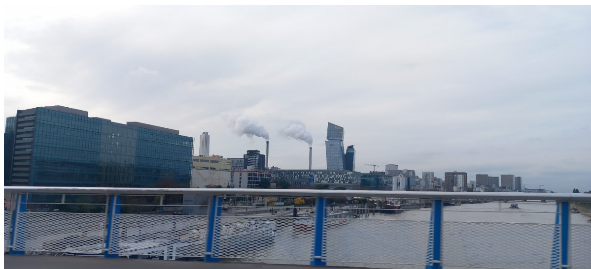
Figure 1: View of the incinerator Ivry-Paris XIII
