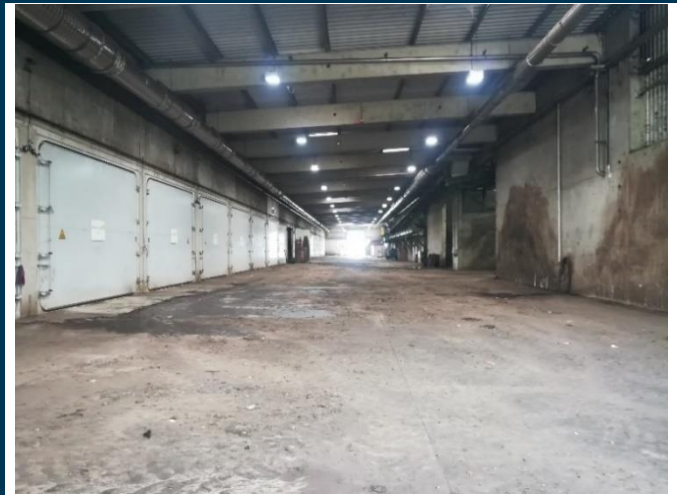
Dry anaerobic digester boxes (Walk, 2019)
