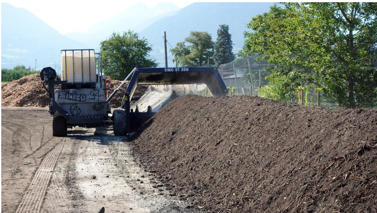
Figure 6. Irrigation on open windrow composting pile
