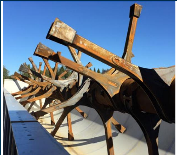
Plug-flow digester under construction (Wilken, 2019)
