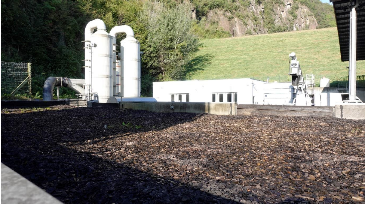
Figure 7. Biofilter for the removal of fumes during enclosed composting
