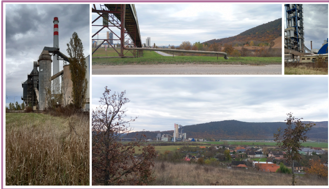
Figure 1 - The cement kiln Turňa nad Bodvou
