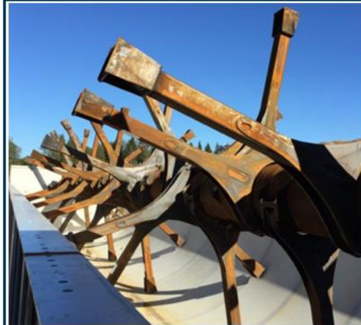
Plug-flow digester under construction (Wilken, 2019)
