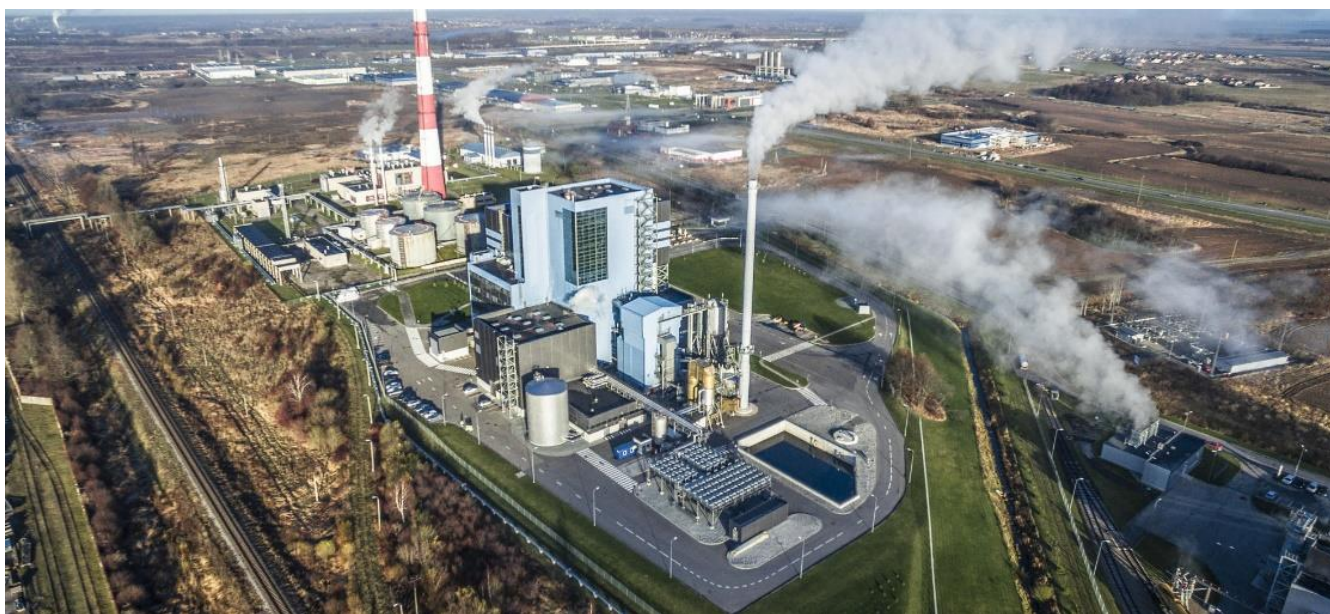
Figure 1. “Fortum Klaipėda” waste incineration plant from bird’s view. Source: “Fortum Klaipėda”
